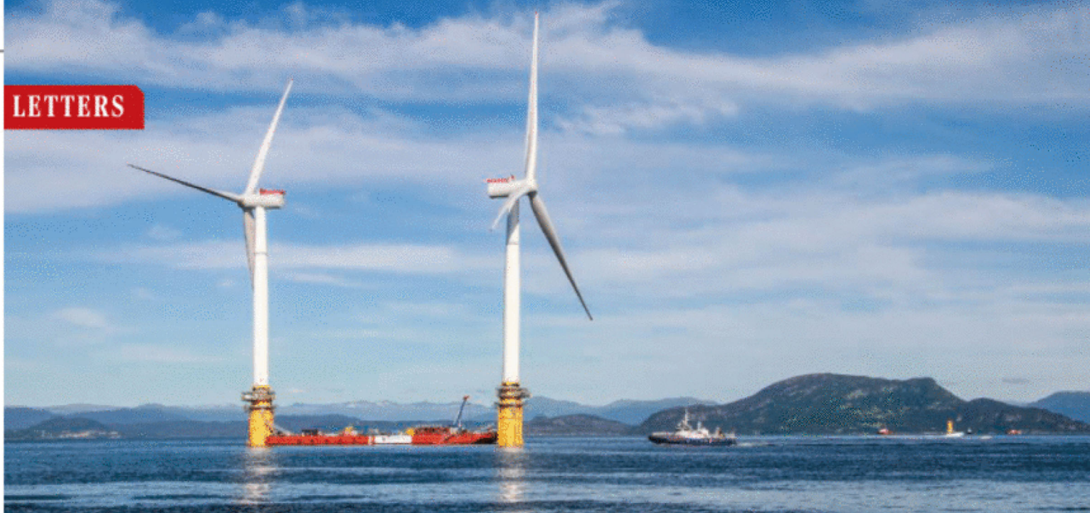
Floating wind turbines, such as these two en route to the world's first floating wind farm, could affect the environment in ways that have not yet been identified.
